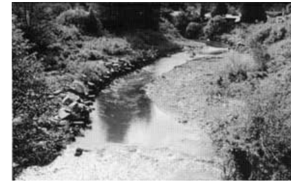
Wolf Creek Phase III after the spring 1995 floods. The rock wier at the bottom of the photo is slowing down the Creek's waters and dissipating erosive energy.
