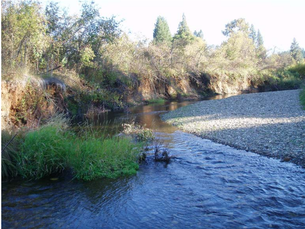
Pre-construction Streambank and Point Bar ( looking upstream from bottom of project )
