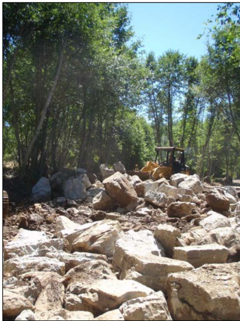
Moving rock and fill for fish passage structure.
